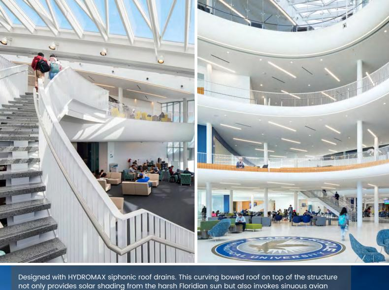
Designed with HYDROMAX siphonic roof drains. This curving bowed roof on top of the structure not only provides solar shading from the harsh Floridian sun but also invokes sinuous avian forms. The vertical, exposed struts convey a feather-like quality and are structural members that tie down the curved roof form from wind uplift, particularly, for hurricane resistance.
